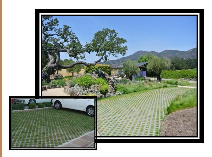
Permeable pavers help rainwater reach the ground. Permeable pavers, such as our Grass-Eco pavers direct water around the surface. The purpose is to ensure stormwater can penetrate the ground rather than flow to municipal drains, retention ponds, or public waterways.
